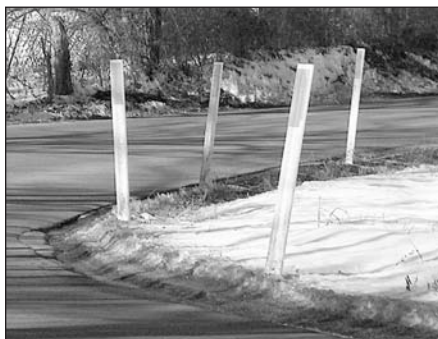
GREENLINE MARKERS IN USE ON INSIDE OF CURVE FOR SNOW PLOWING LOCATION
